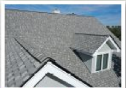
You get a brand new roof at little to no cost to you!
