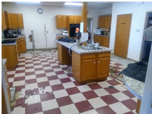
Starting to remove old flooring
