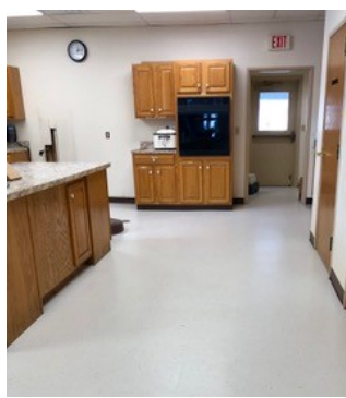
floor installed-not waxed
