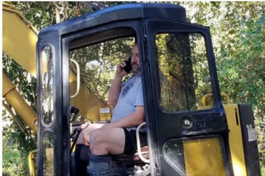
Lake's own resident and community asset, Mason Crafters, and at the helm of the shovel is Tony Sartori.
