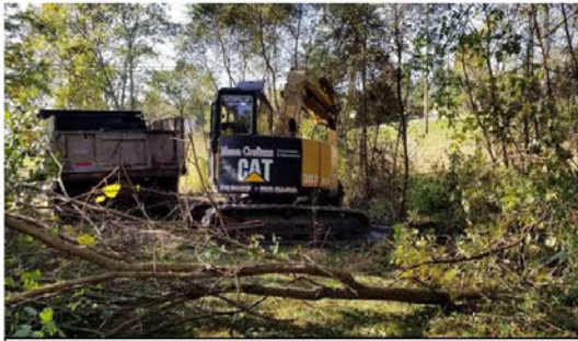
Work in progress as the big shovel removes the muck from the bottom behind cleared brush in the foreground.
