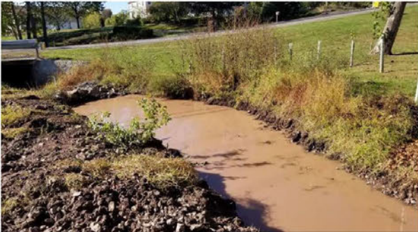
Rejuvenated portion just off the road...wider, silt's gone, and the small and larger rock (out of view) dams reconstructed.
