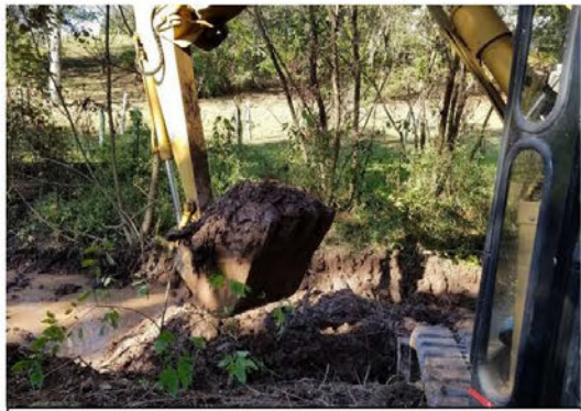
Closer view of a section of creek being completed.
